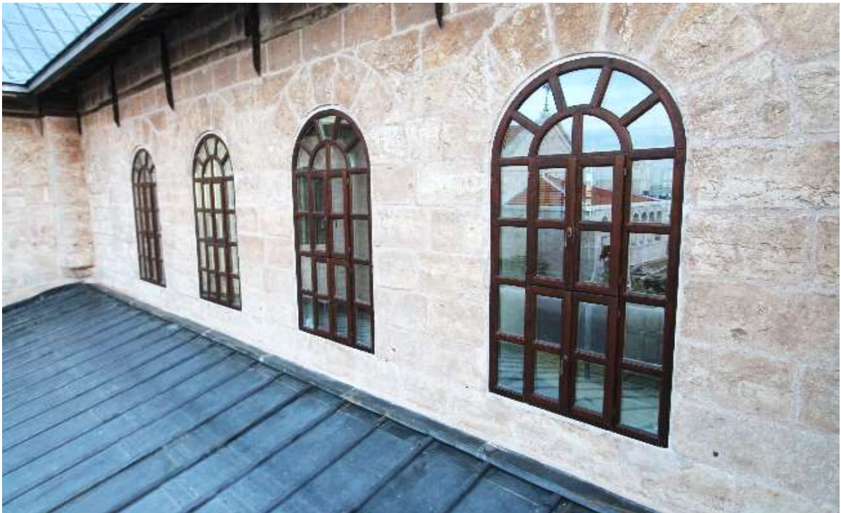
The new wooden windows
