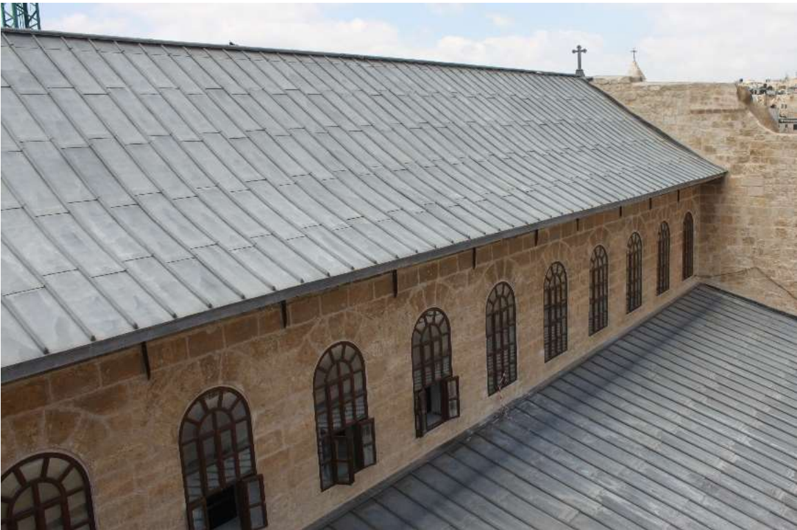
The lead roof before and after restoration
