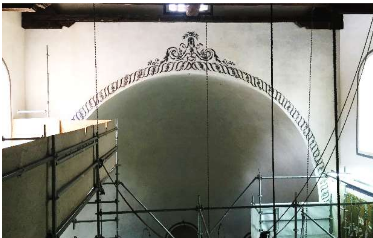
The internal plastering surfaces after restoration
