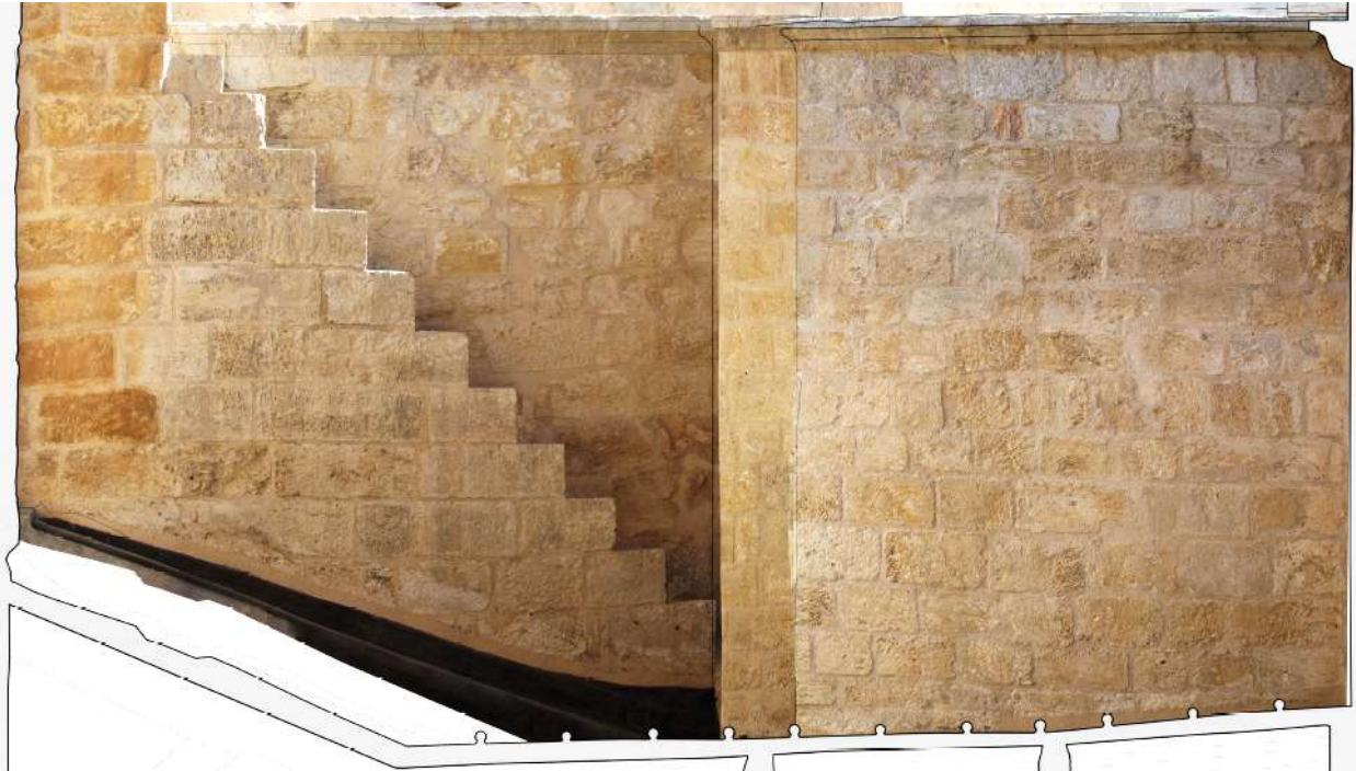
Northern corner – After restoration
