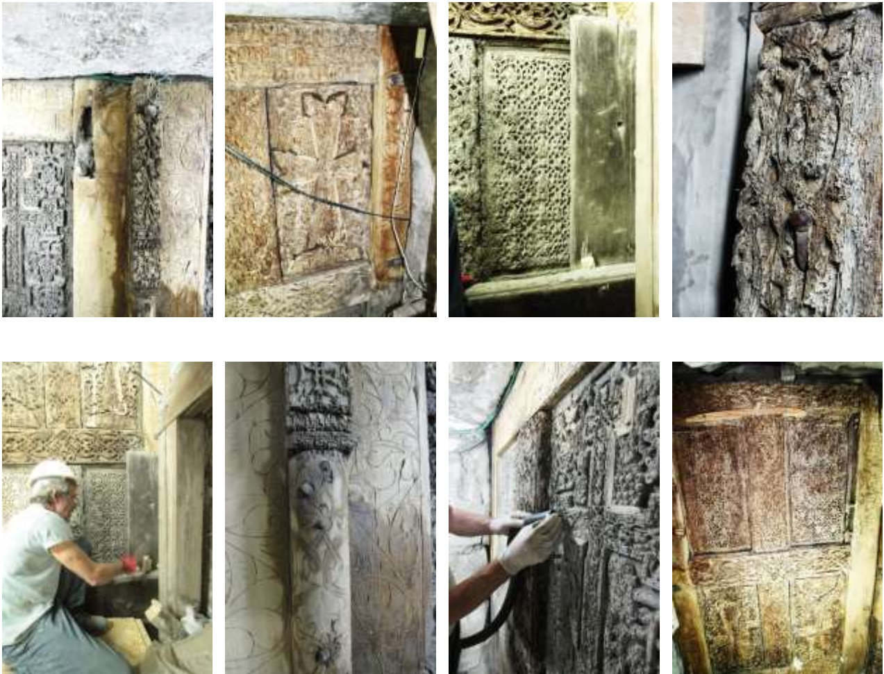
The Narthex eastern door during the restoration works
