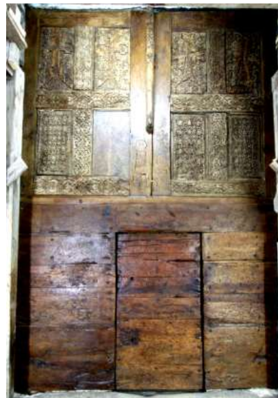
Narthex wooden door after restoration
