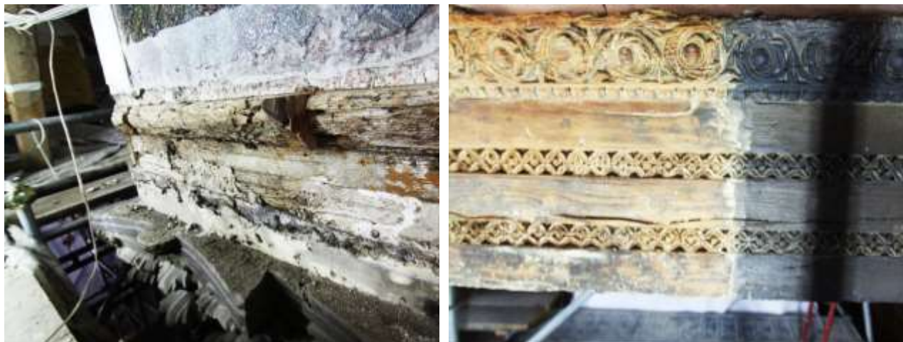
The wooden Architraves before restoration
