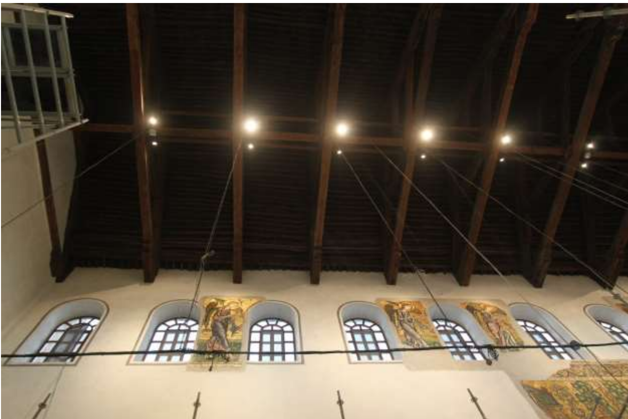
The new lighting system at the central nave
